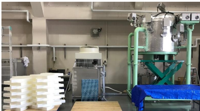
Tray for lees Cooling system Distillation equipment
