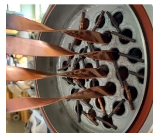
Condenser turbofin (copper)
